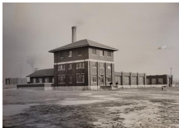
City of Monroe Water Plant – In service since March 1, 1924
